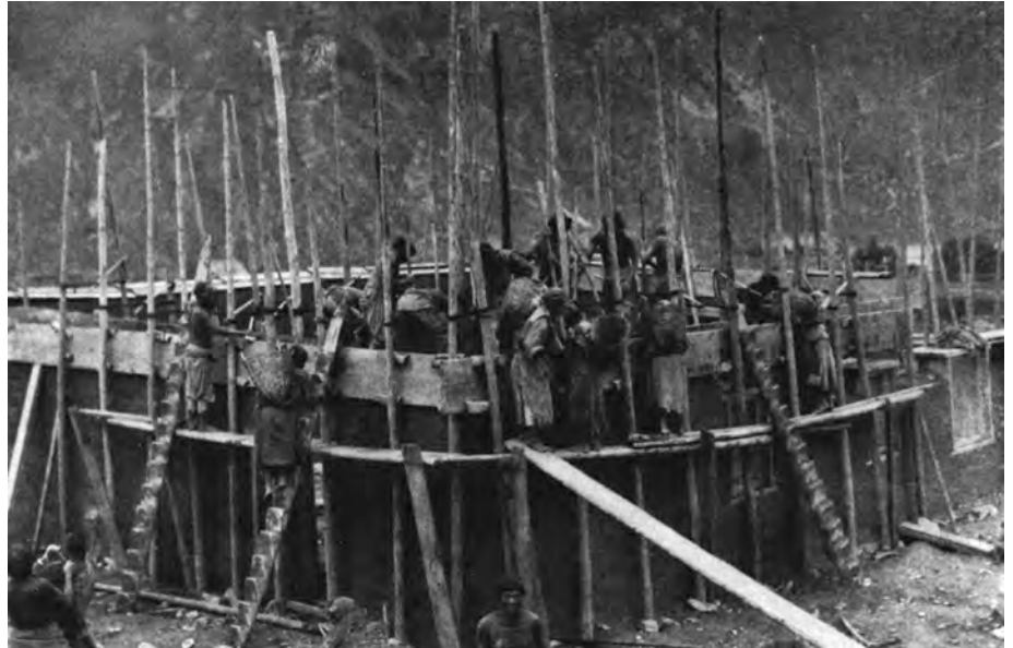
(Below) House under construction showing the notched poles used as ladders throughout Tibet
